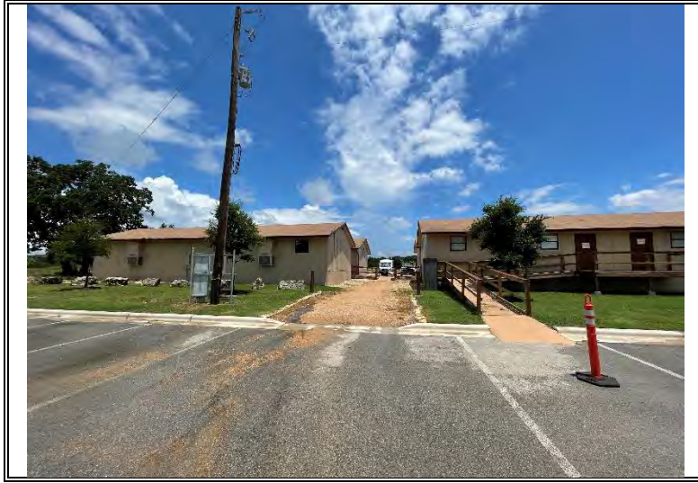
Modular buildings in area of acquisition
