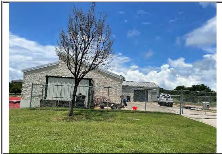
Maintenance building (not impacted)
